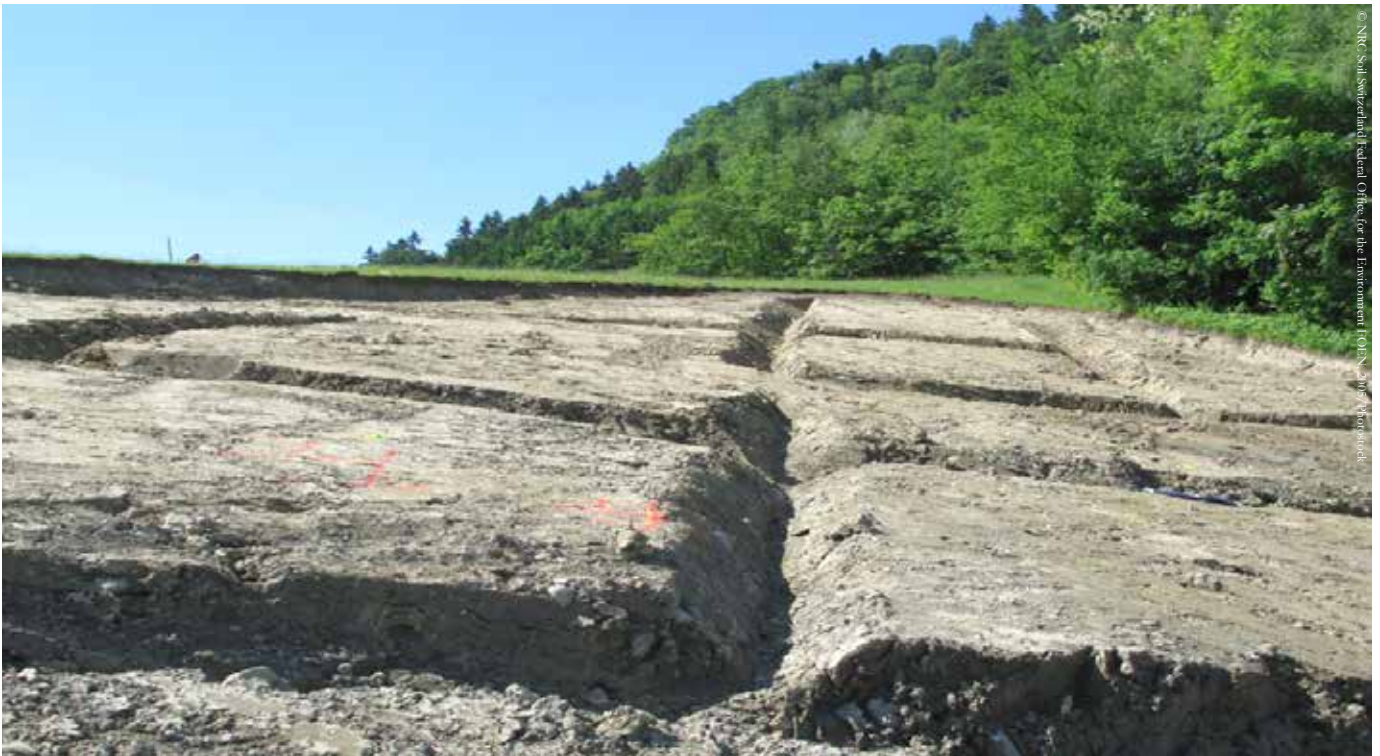
Construction of surface drainage features for controlled management of the rainwater
