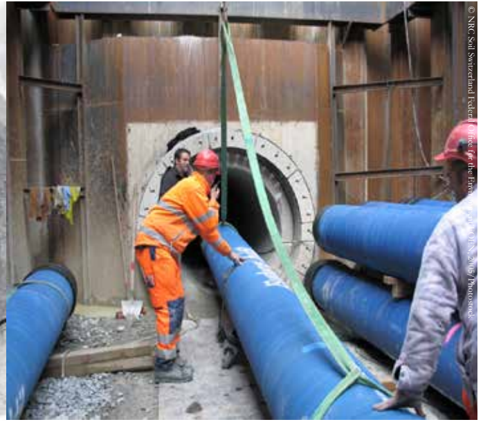
Introduction of the new drinking-water pipe into the diverted channel
