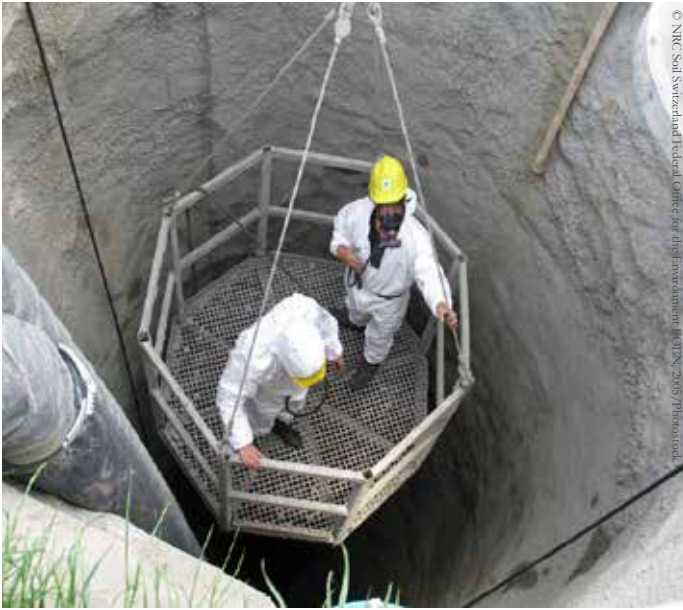
Channel for construction of the new base drainage system
