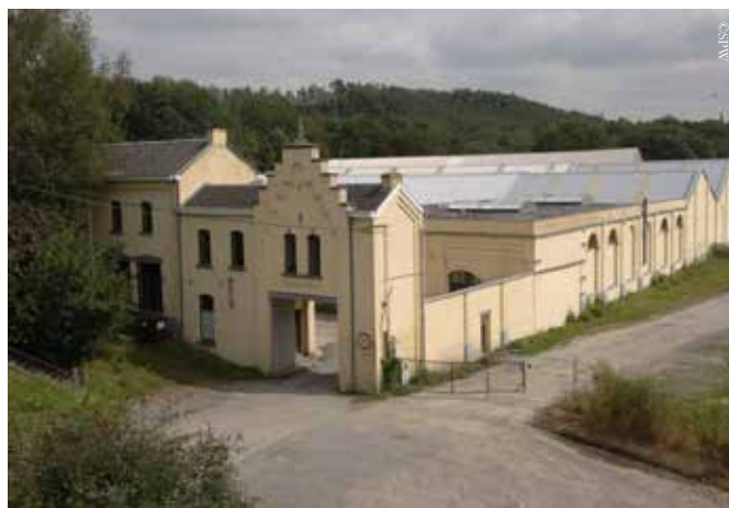
Ancient bolt factory, located in Morlanwelz, rehabilitated in sports hall, offices, youth center (sports and social activities)
