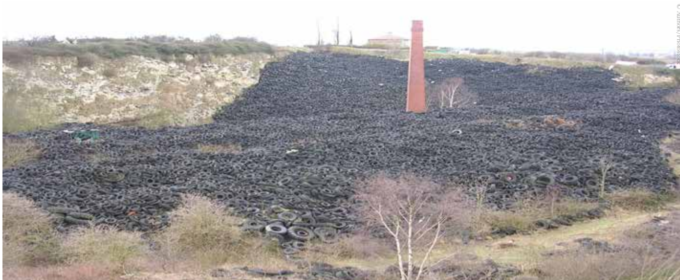
The quarry before any remedial works
