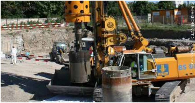
Austria. Large diameter boreholes and steel piling coffer
