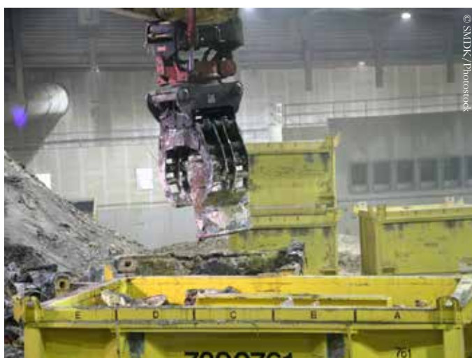
Retrieving a waste drum with the excavator.
