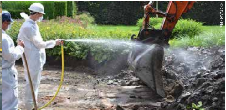
Belgium. Large-scale asbestos remediation works
