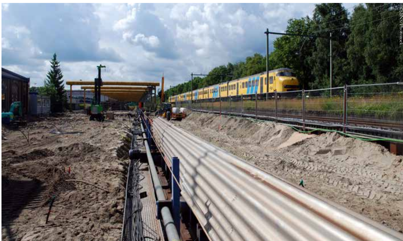
Site of remediation along the railway line.
