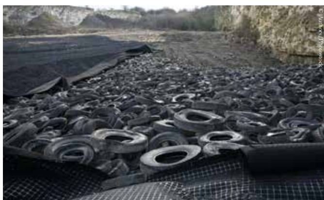
From left to right: Laying the geogrid membrane.. Removal and recycling of tyres
