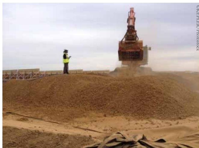
Soil turning and applying of the solution of nutrients and microorganisms.
