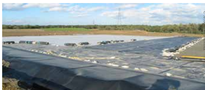
Bois Saint-Jean, Belgium remediation works
