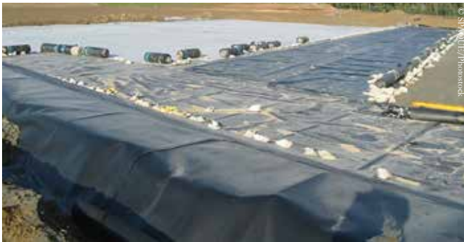
Belgium, Bois Saint-Jean. Remediation works
