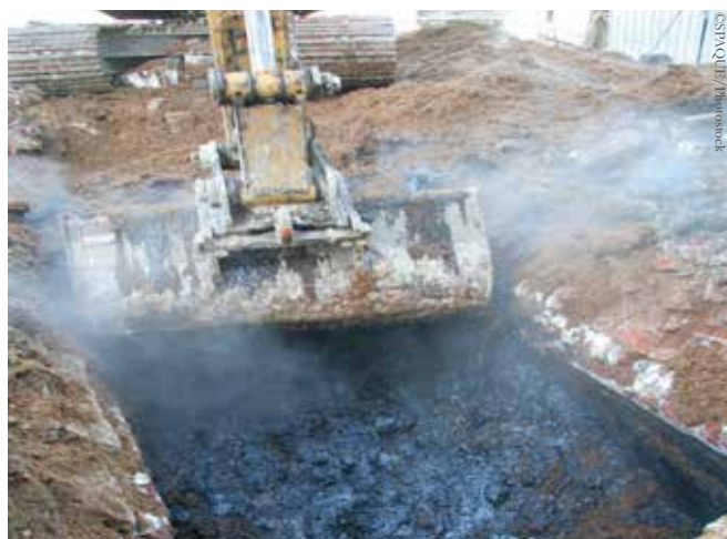
Old gasworks-site and remediation works in Mons, Belgium
