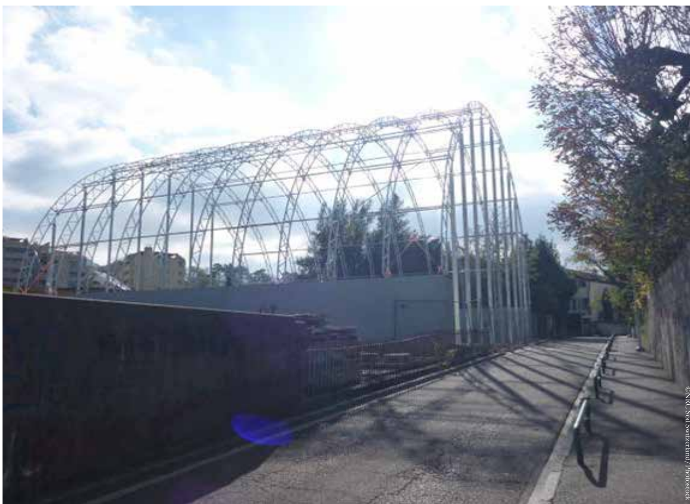
Protective cover under construction
