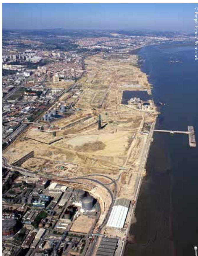
Aerial view of earthworks at Park of Nations
