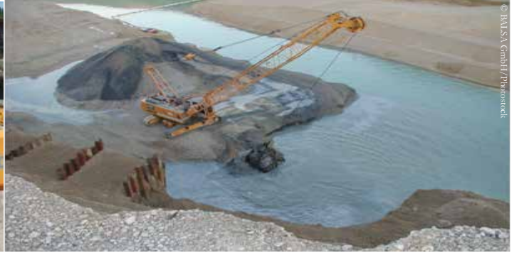
Austria. Excavation of the contaminated sediments below groundwater table
