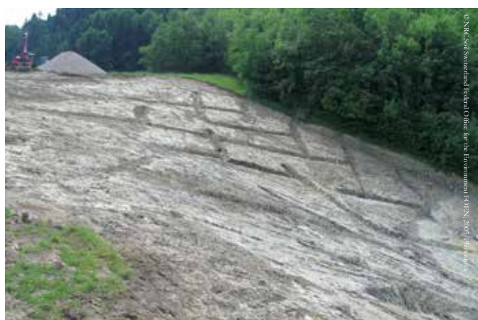
Construction of surface drainage features for controlled management of the rainwater.
