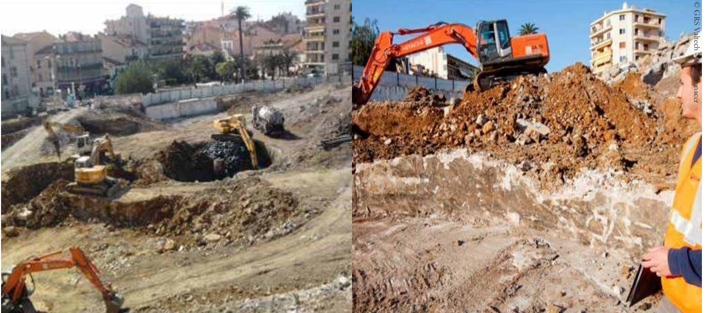
France, Cannes. Remediation works at former GDF-Suez gas plant
