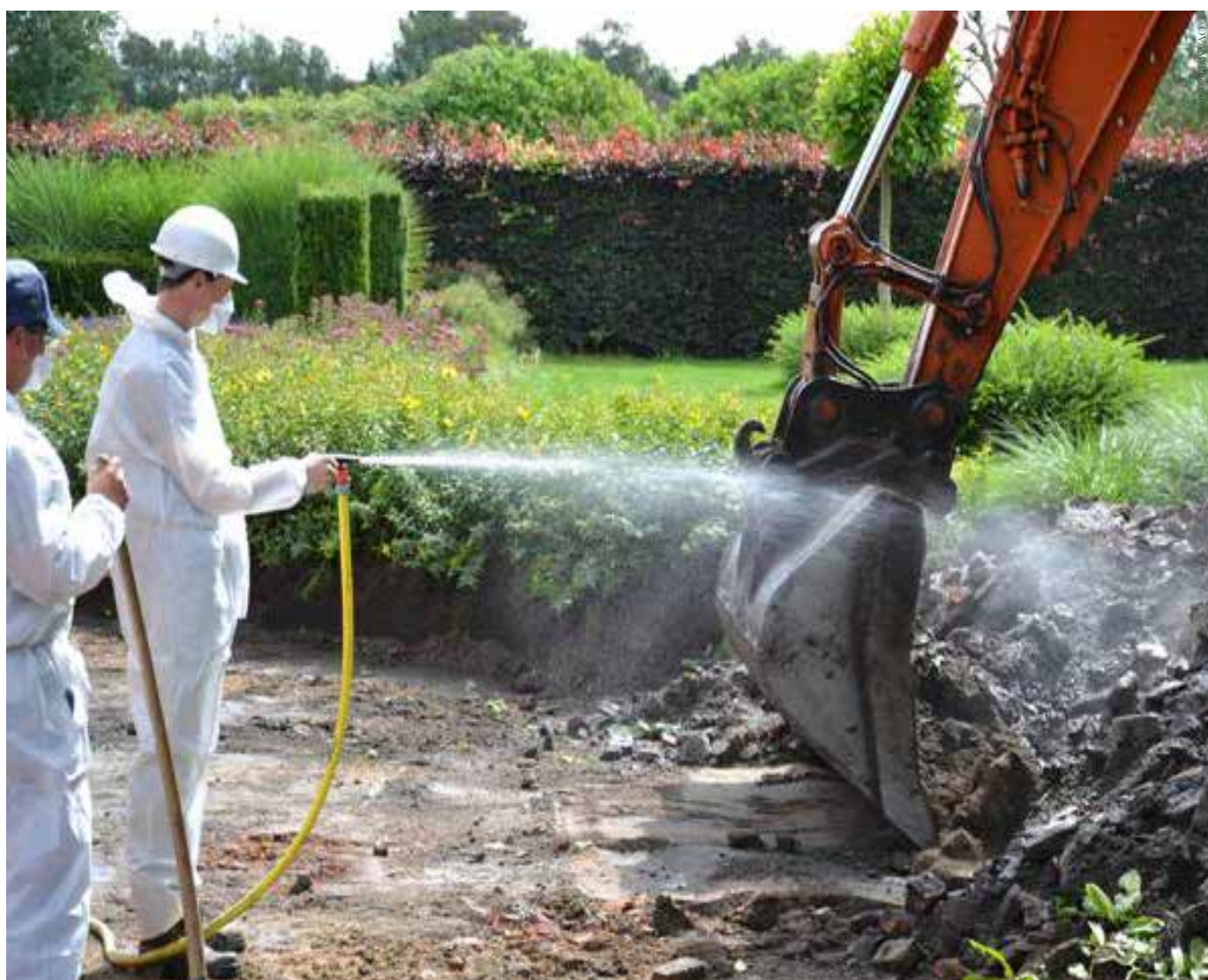
Workers removing asbestos
